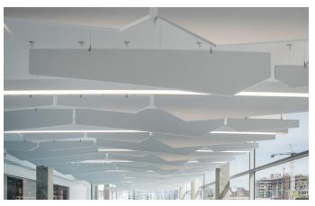
Built-in features designed to reduce echoes and improve sound absorption, include ceiling tiles, wall panels, and acoustic baffles.
